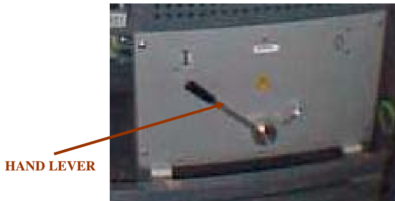
Figure 6.8 Disconnecting and Earthing Device
