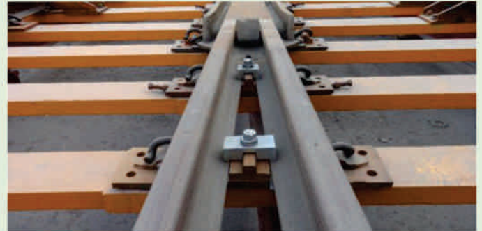
Figure 2 Weldable CMS crossing
