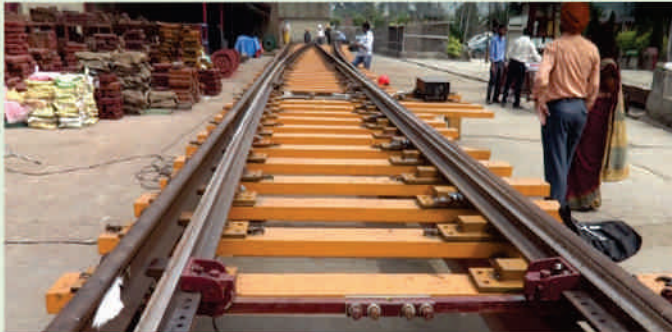
Figure 1 View of 1 in 12 canted turnout
