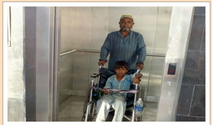
Lifts installed at Dwarka
