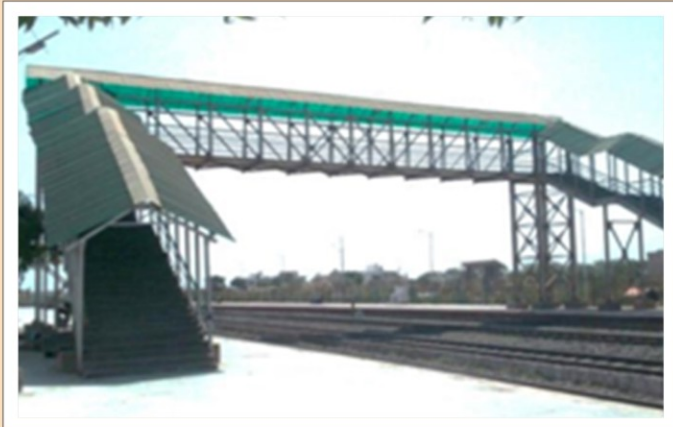
New Foot Over Bridge at Adipur station
