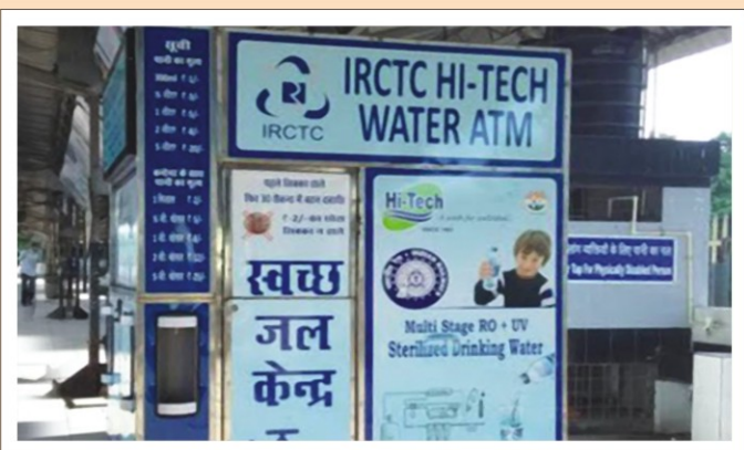
Water Vending Machine installed at stations
