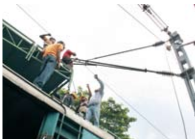
Over Head Electrical maintenance, South Eastern Railway.
