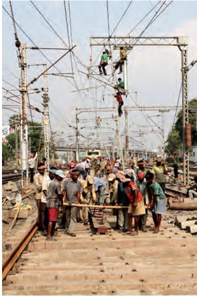
OHE erection and installation of Diamond Crossing, South Eastern Railway
