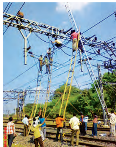
DC-AC conversion work in progress on Central Railway
