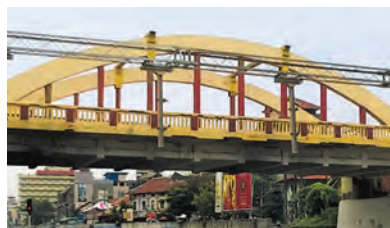
Lifting of ROB for OHE underneath by CORE
