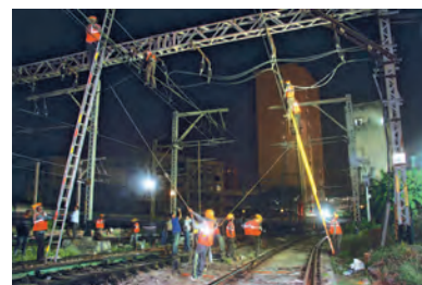
Test Charging of DC-AC Conversion, CR
