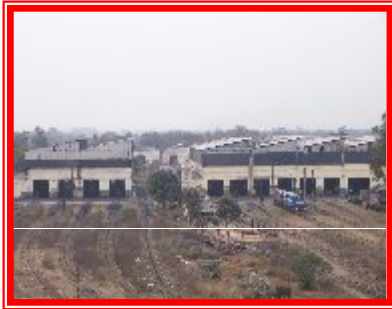
Photo of Shed
