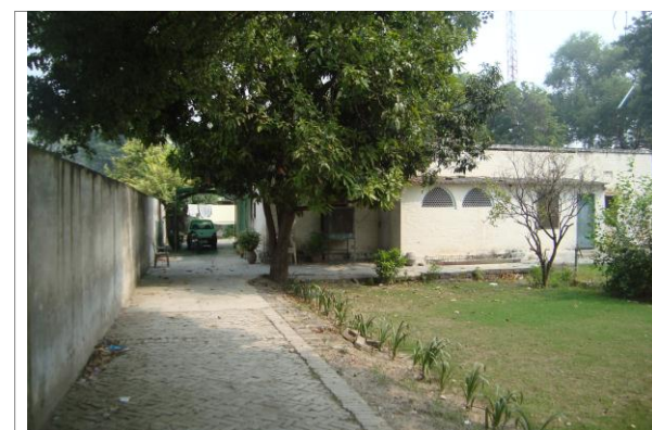
Photo 5: Site picture showing the quarters to be dismantled
