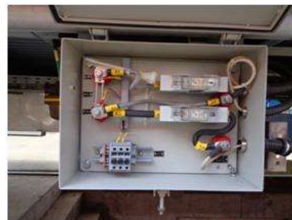
Figure 1.15 : Battery Fuse Box (-ve)
