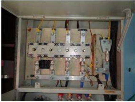
Figure 1.34 Rotary Junction Box
