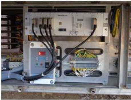
Figure 1.20 Pump controller
