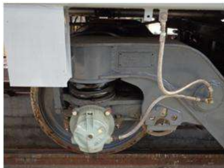
Figure 1.18 Wheel set and earthing equipment
