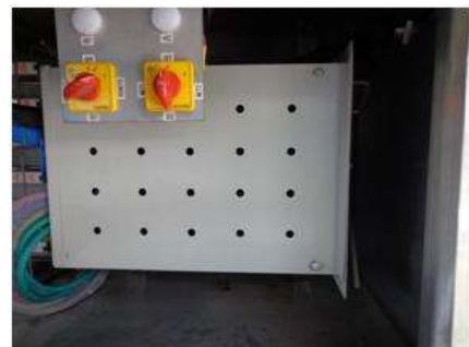
Figure 1.5 Disconnecting and Earthing Device
