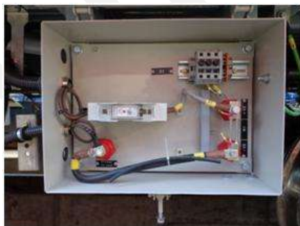
Figure 1.14 : Battery Fuse Box (+ve)
