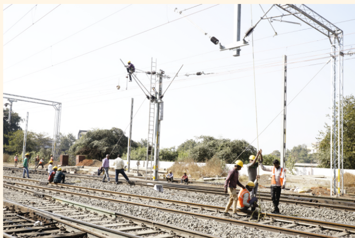
Electrification work between Itarsi - Jabalpur section
