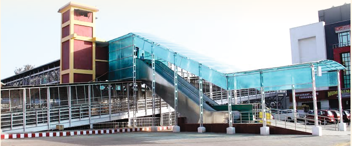
Escalator at Jabalpur Station
