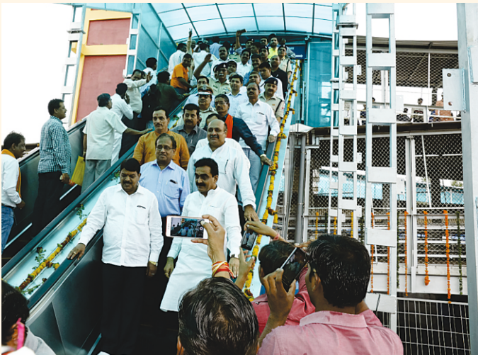
Escalator at Jabalpur station
