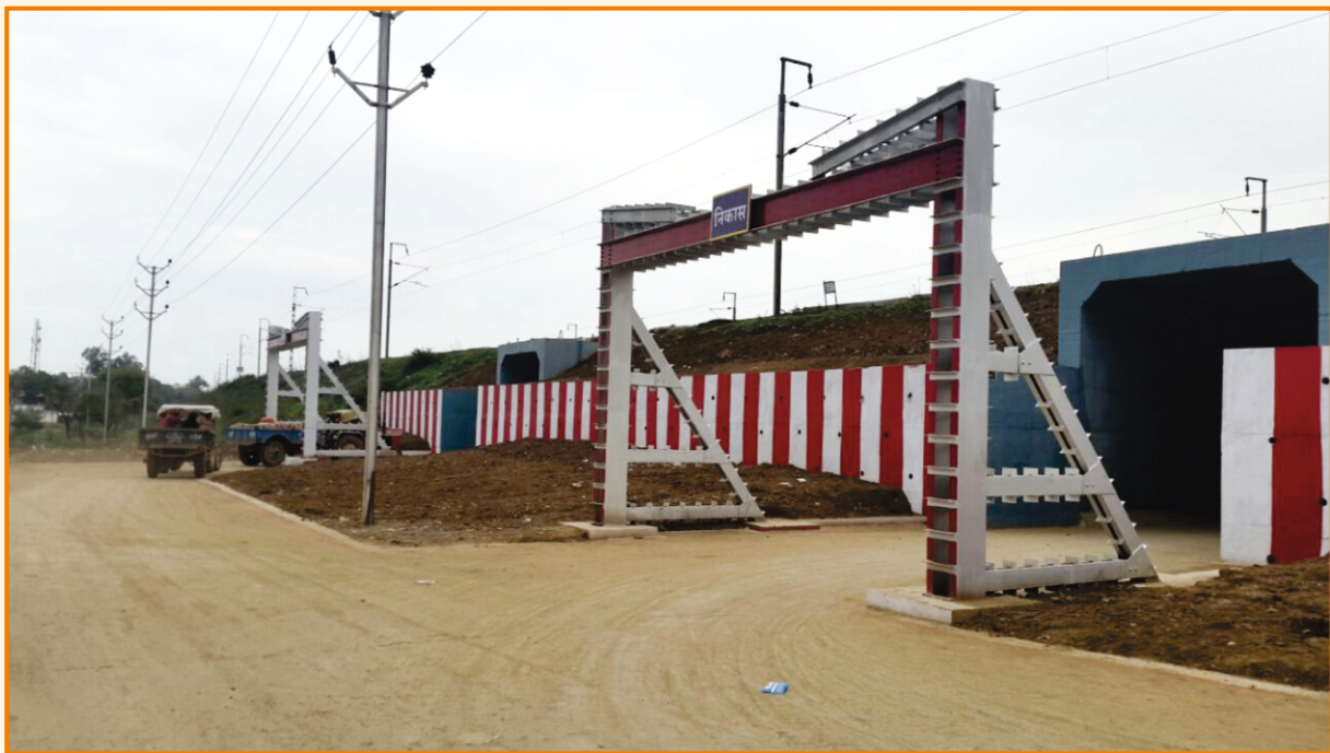
Railway Under Bridge at Katni Murwara
