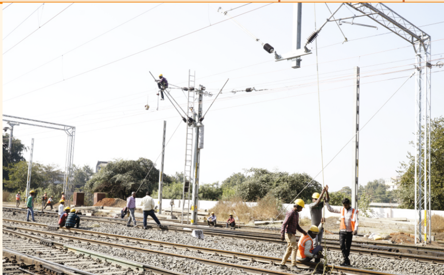
Electrification work at Jabalpur yard
