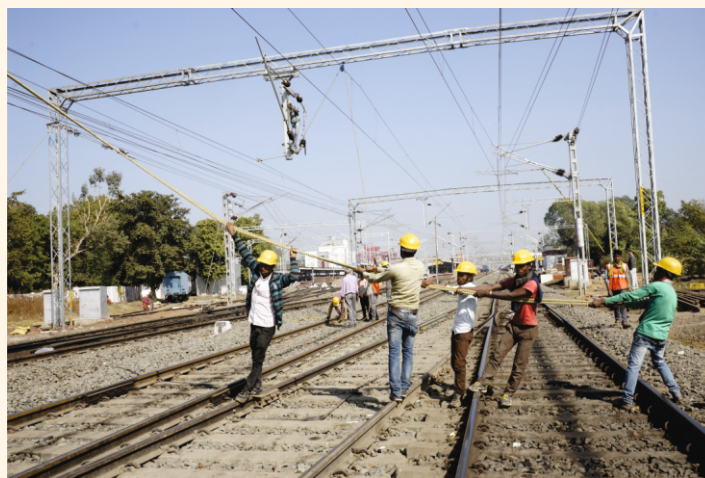
Electrification work between Itarsi - Jabalpur section
