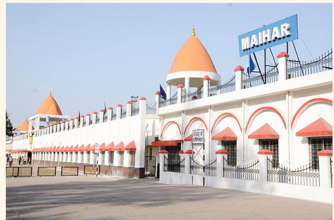
Clean Station - Maihar
