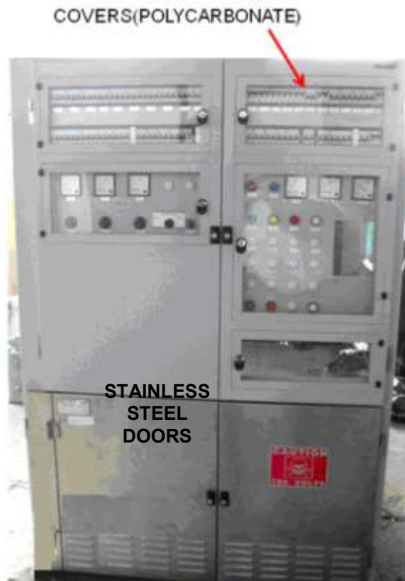
Figure 6.7 Modified Doors Arrangement
