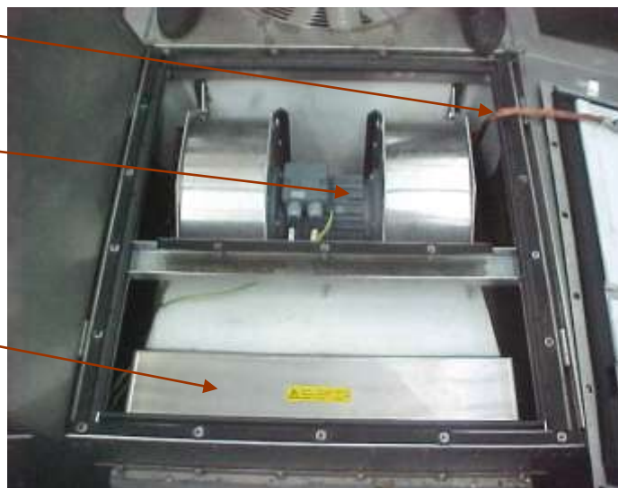
Figure 6.11 Evaporator Motor Unit in RMPU
