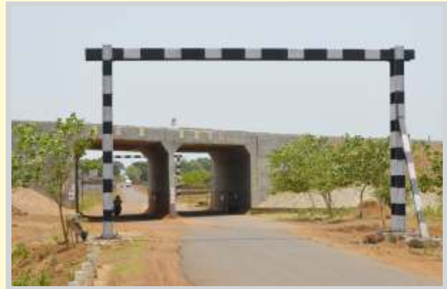
Road Under Bridge near Khurda Town Station
