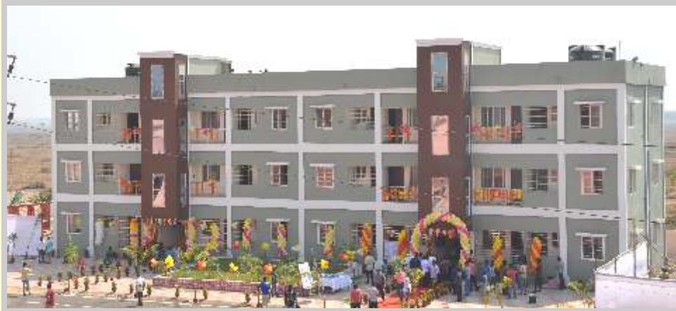
Pre-Fabricated Residential Building at Jakhapura
