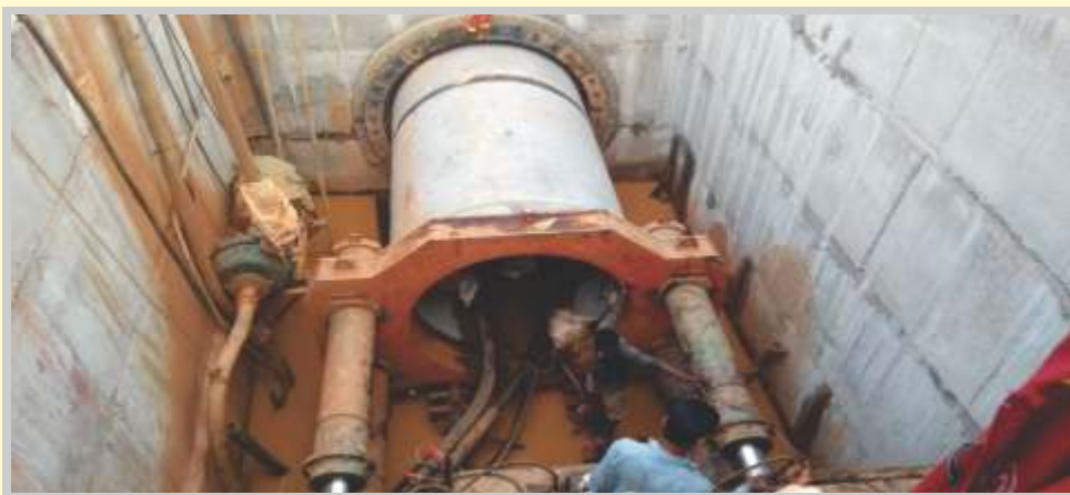
Micro-Tunnelling process in progress at Bhubaneswar Station
