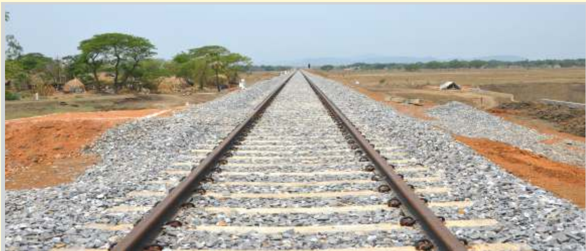
New Line between Khurda Road and Nayagarh Town
