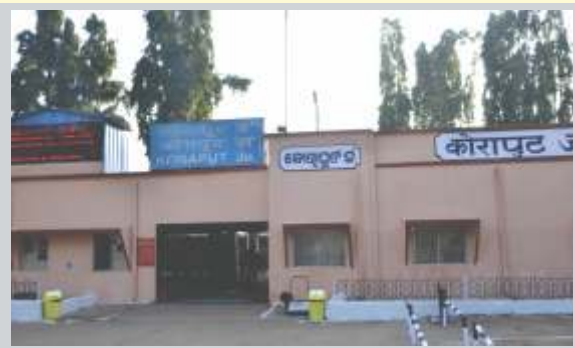
Koraput Station to be developed as Adarsh Station
