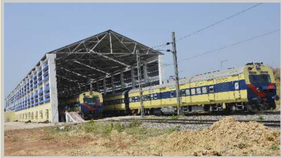
Newly constructed MEMU Shed at Khurda Road
