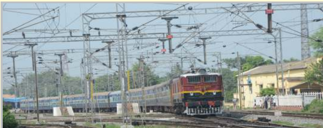
Electrified Train Route near Cuttack Station
