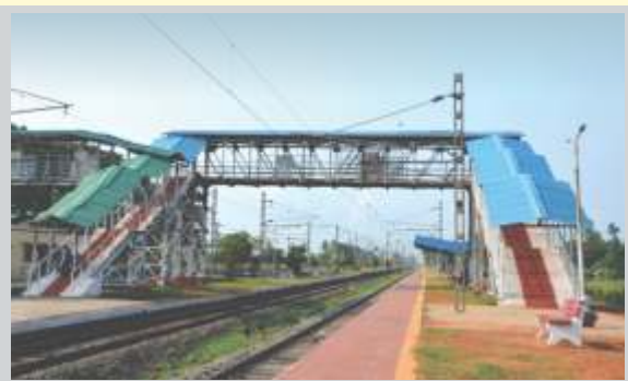
Foot Over Bridge at Sakhigopal
