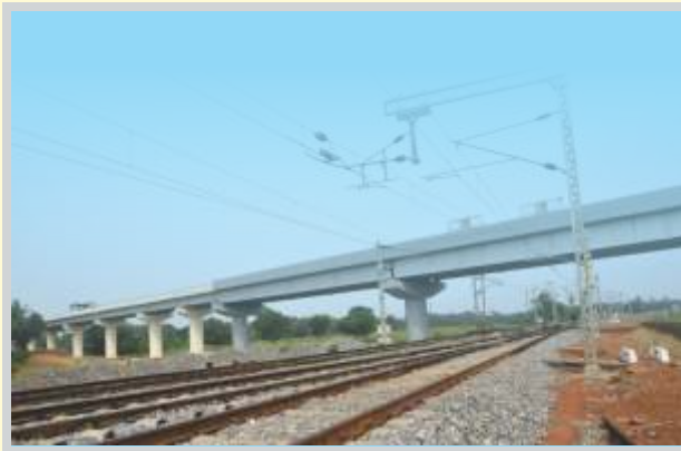
Road Over Bridge at Malatipatpur
